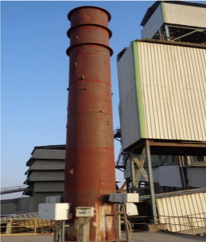
CEMS in the stack of Bag House of Cement Mill-3, Imlai
