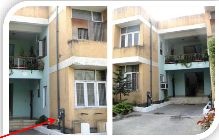
RWH Filter at Sr Block Colony at Narsingarh
