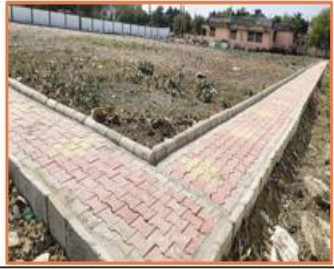
Installation of Paver Blocks in District Ayush Center @ Damoh
