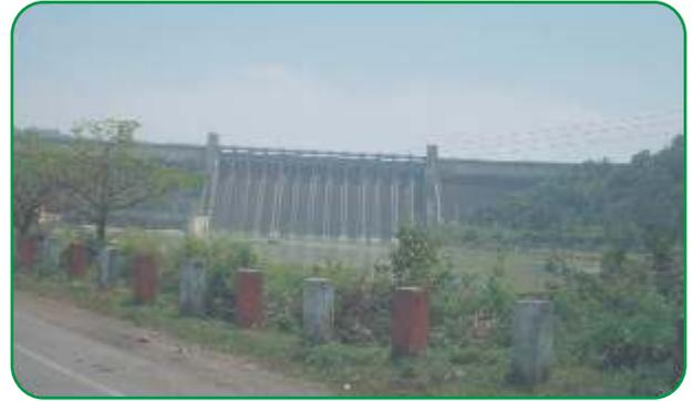
Metturu Dam Mysore constructed by using Fly Ash
