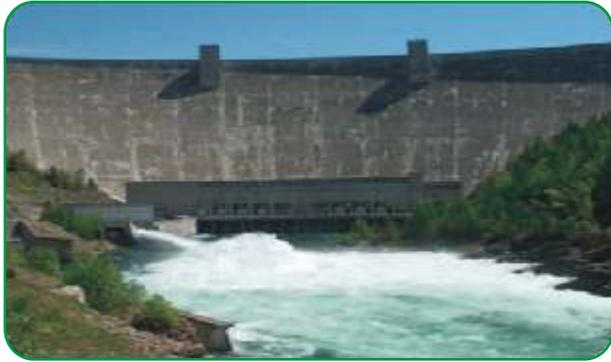
Hungary Horse Dam constructed by using Fly Ash
