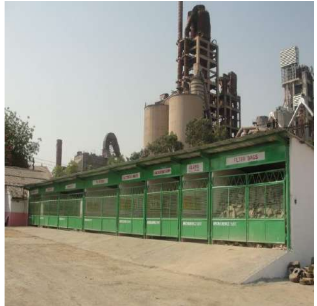
Separate Storage yard for different type of waste such as filter bag, Glass, Used Batteries, E-waste, Turning Metals etc.
