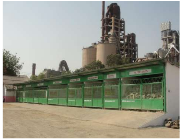
Separate Storage yard for different type of waste such as filter bag, Glass, Used Batteries, E-waste, Turning Metals etc.
