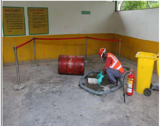
Used Oil and Grease spill trapping, by using all necessary PPEs
