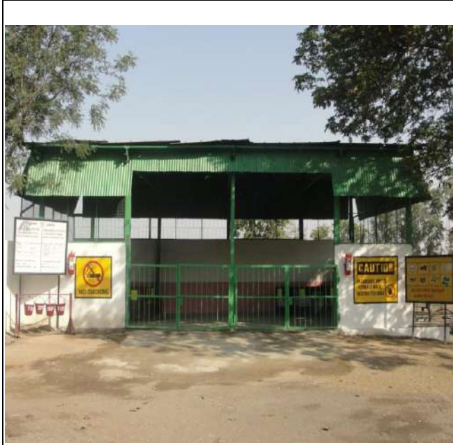
Hazardous waste Storage Yard for Category 5.1 & 5.2 at Clinkerisation Unit – Narsingarh.
