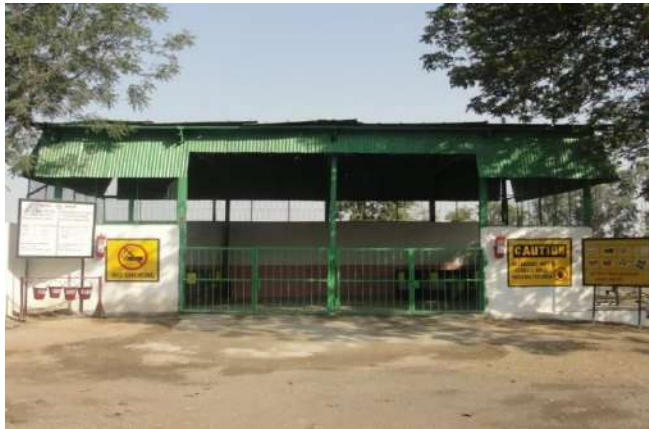
Hazardous waste Storage Yard for Category 5.1 & 5.2 at Clinkerisation Unit – Narsingarh.
