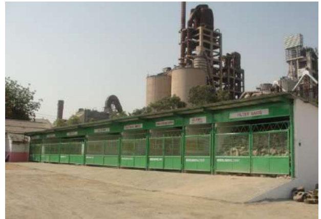
Separate Storage yard for different type of waste such as filter bag, Glass, Used Batteries, E-waste, Turning Metals etc.
