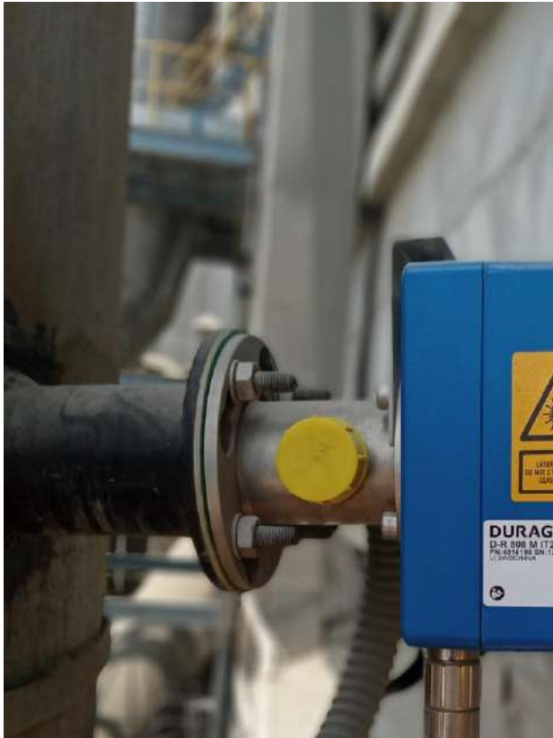
CEMS in Ball Mill Bag House Stack
